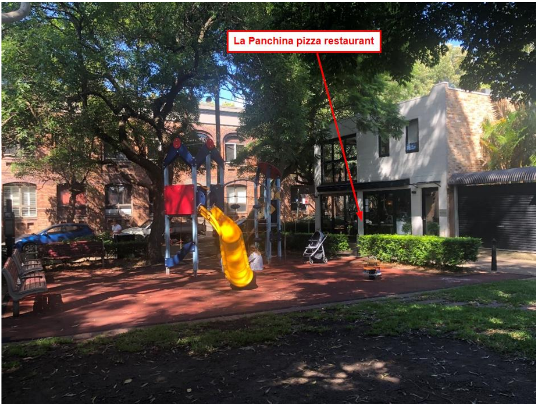
Existing playground in the reserve looking south towards Arthur Street – play equipment is at the end of its lifecycle; soft-fall is worn and separating from edges. Playground is well shaded from the existing trees. Small area of turf in poor condition.
