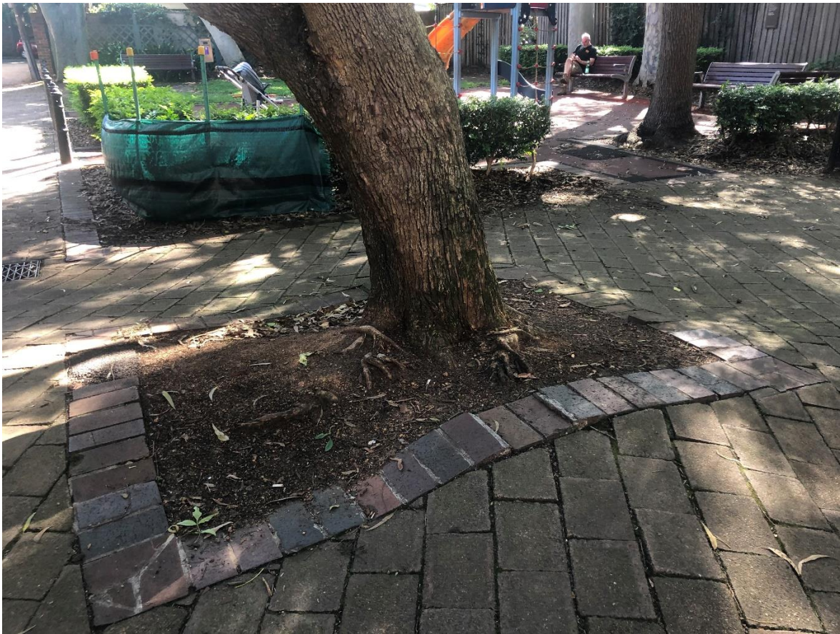
Uneven paving around street tree due to tree roots
